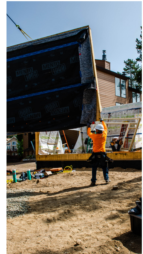
Figure 7: On site panel assembly in Fraser
