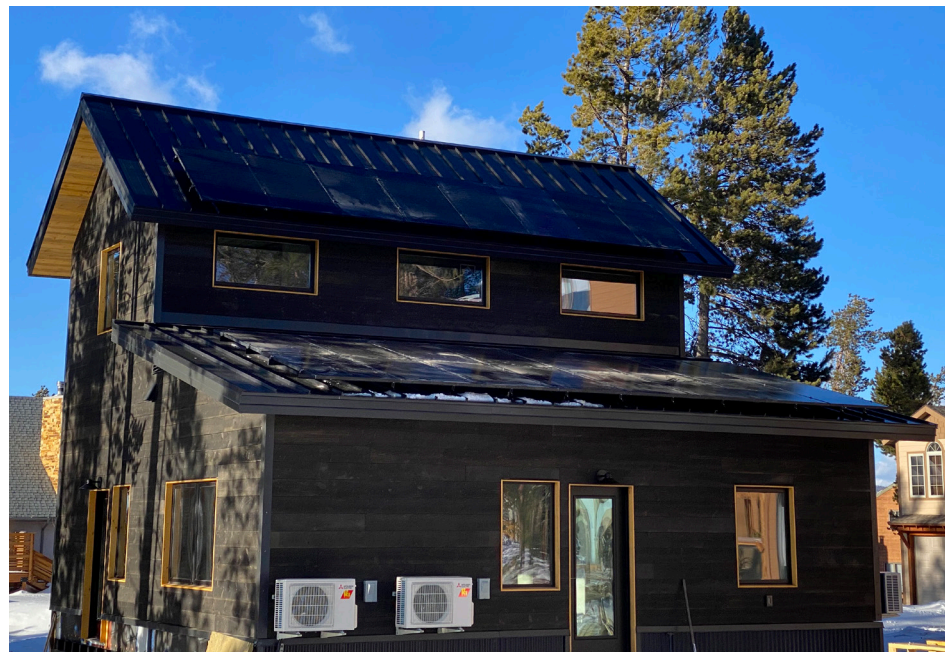
Figure 13: Exterior showing window placement, PV, & 2 of 3 exterior heat pump units
