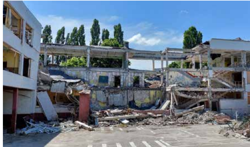
The south wing of Kharkiv School #46 was destroyed beyond repair. The remainder of the school is still intact, with its original concrete post-and-beam construction.
