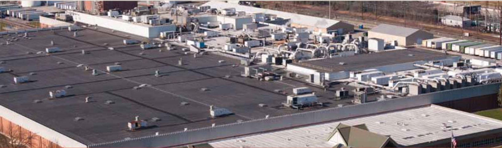
Kellogg Company Plant and Bakery - Lancaster, Pennsylvania
