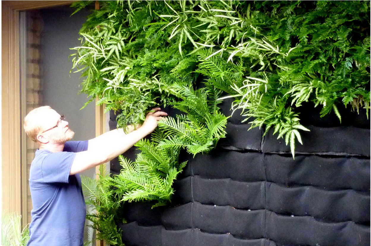
Chris Bribach planting a fully filled in fern wall for a private home in Los Altos Hills, California.
