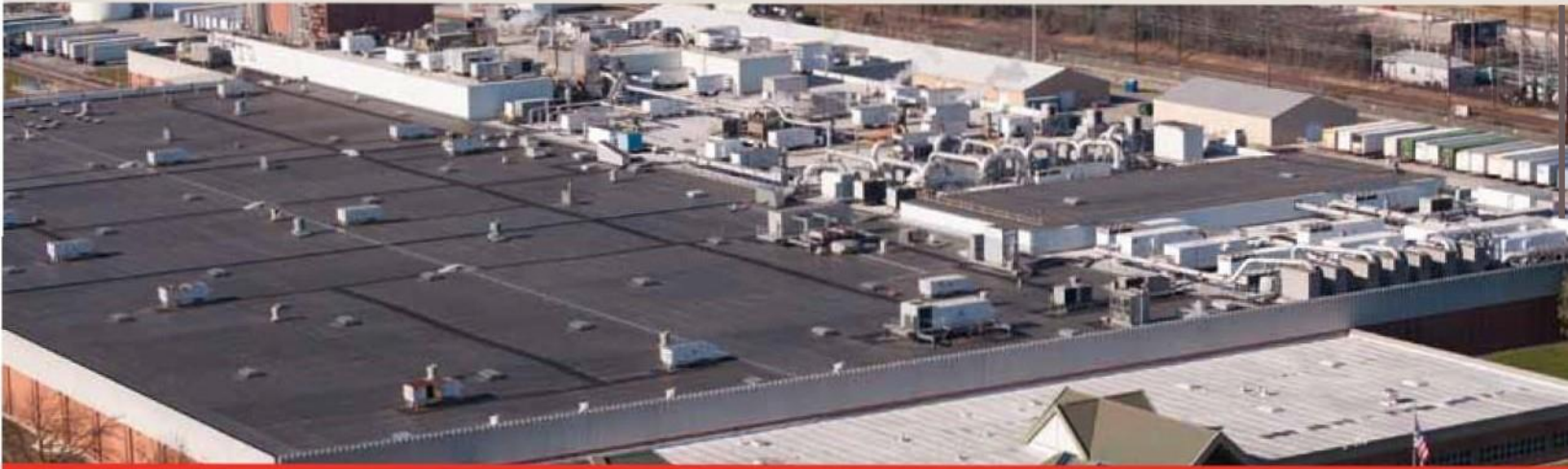
Kellogg Company Plant and Bakery - Lancaster, Pennsylvania
