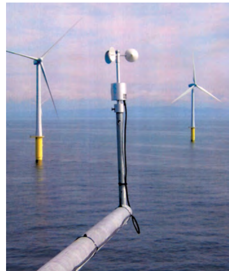
Photo courtesy: rpower renewables
