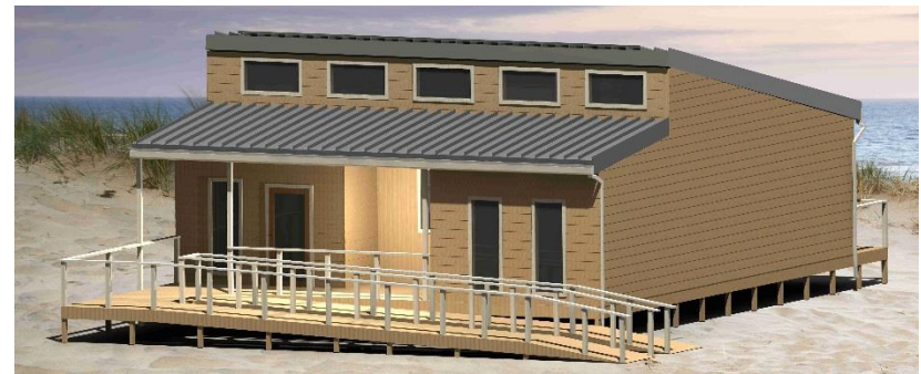
Figure 5: Front Exterior of The BEACH House
