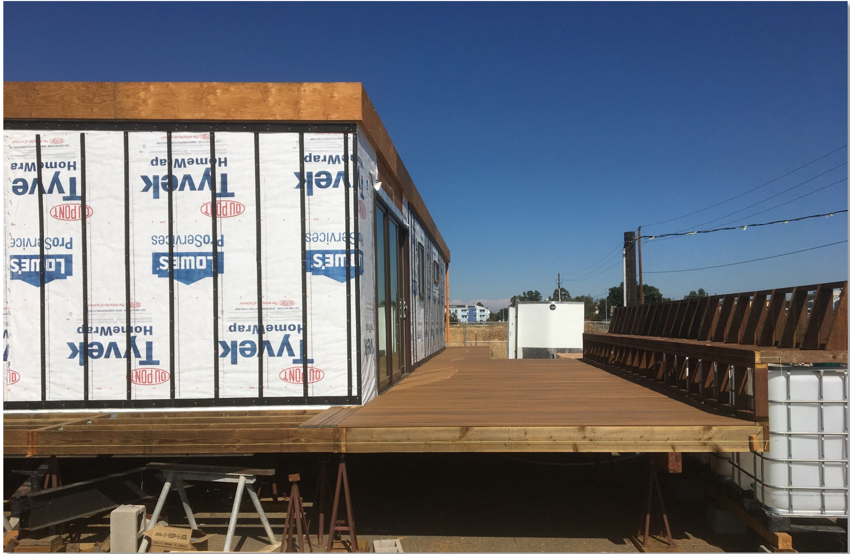
Figure A6: South deck view of bench and IBC structure
