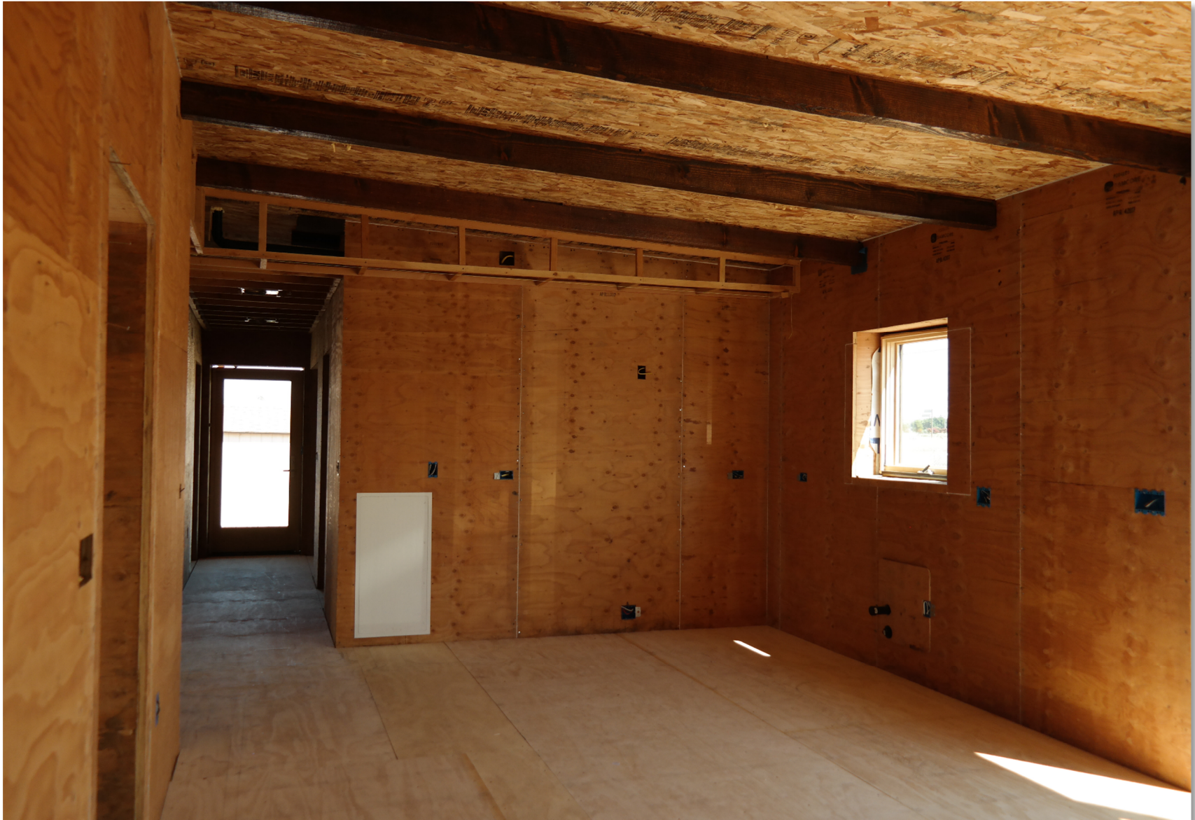
Figure A1: Interior kitchen view facing East
