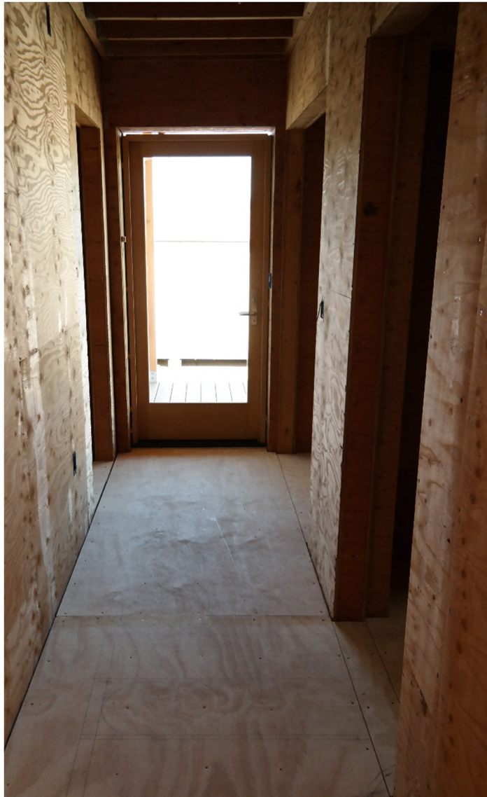
Figure A5: Hallway view
