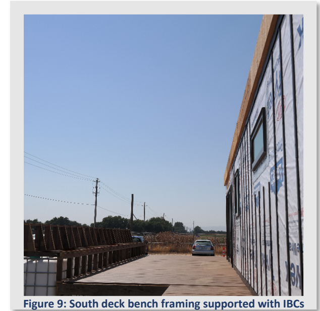
Figure 9: South deck bench framing supported with IBCs
