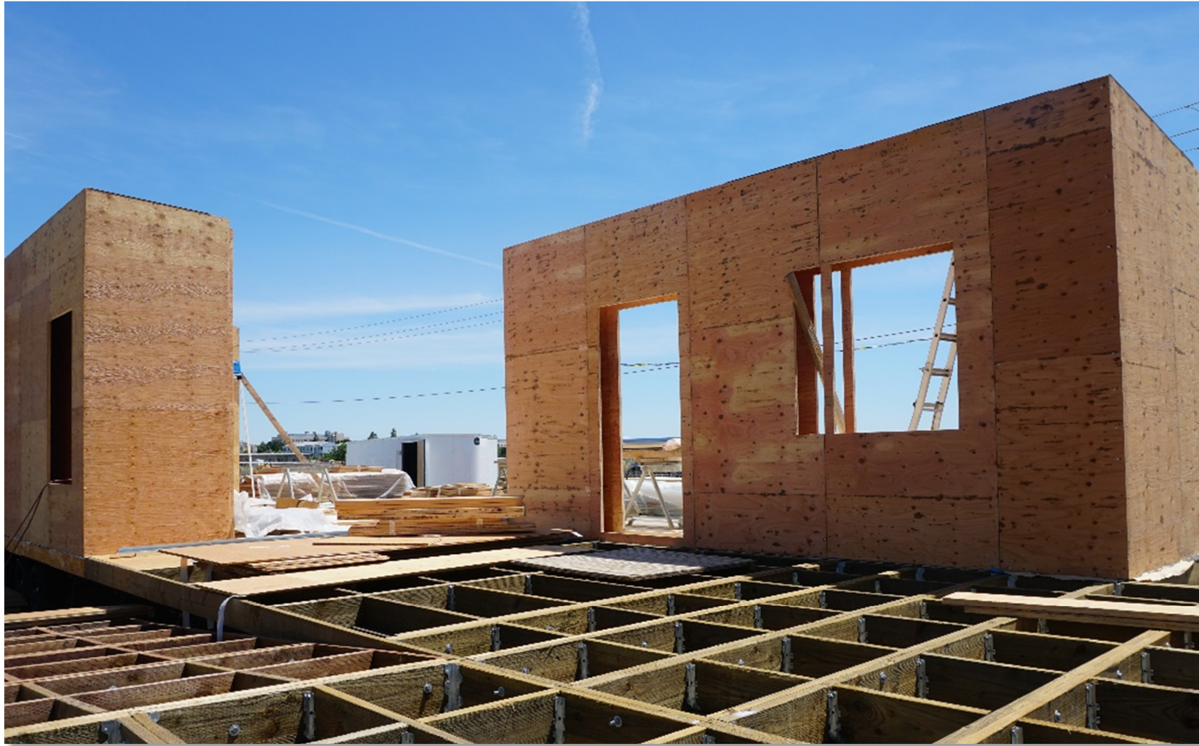
Figure A7: North view of BamCore Wall system installation
