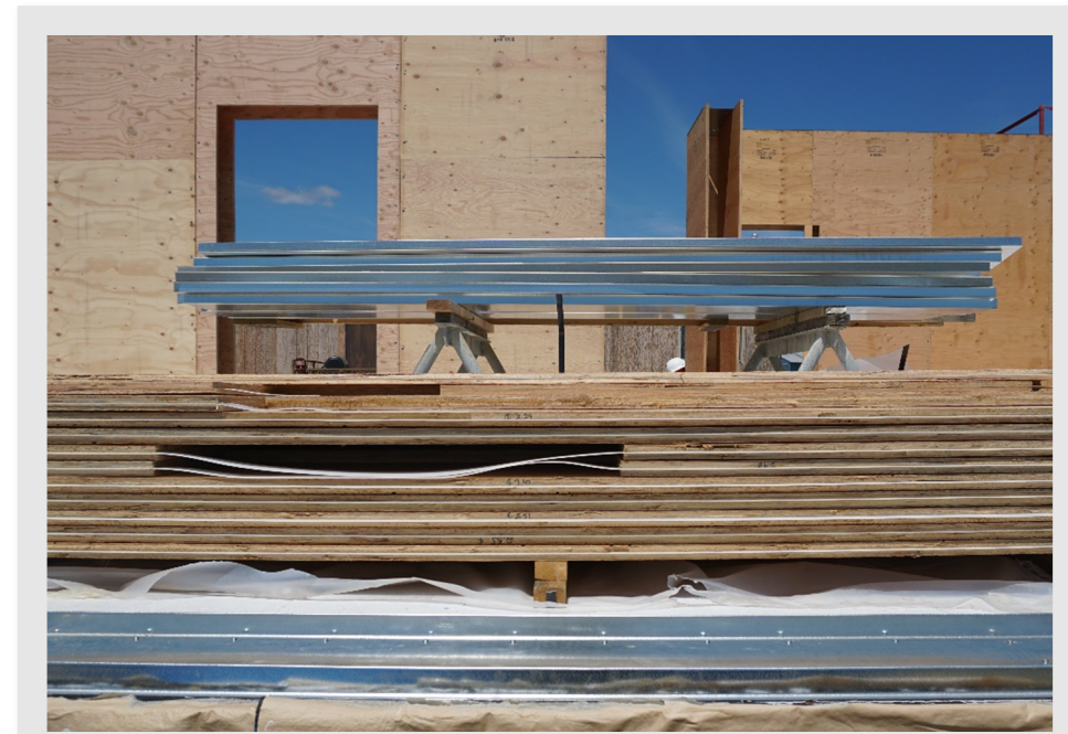
Figure 5: Close-up of BamCore® panelized Prime Wall® System
