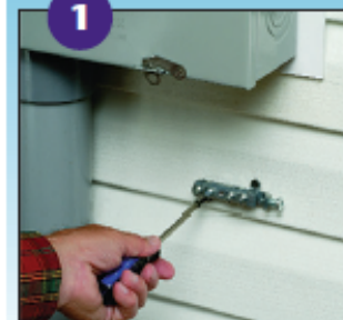
1 Attach grounding bridge to substrate. (Mounting screws not provided.)
