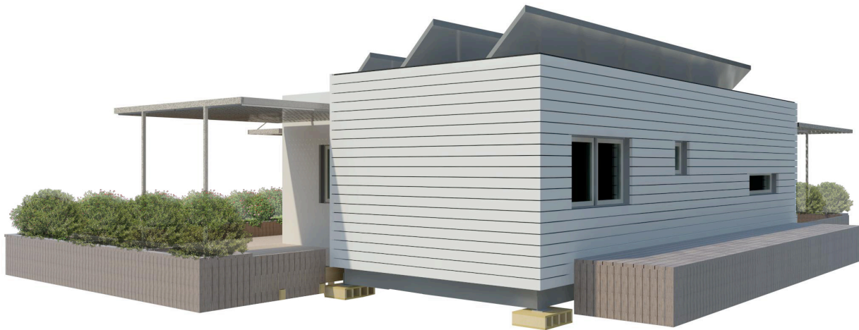
Figure A5: Shading devices on East facade
