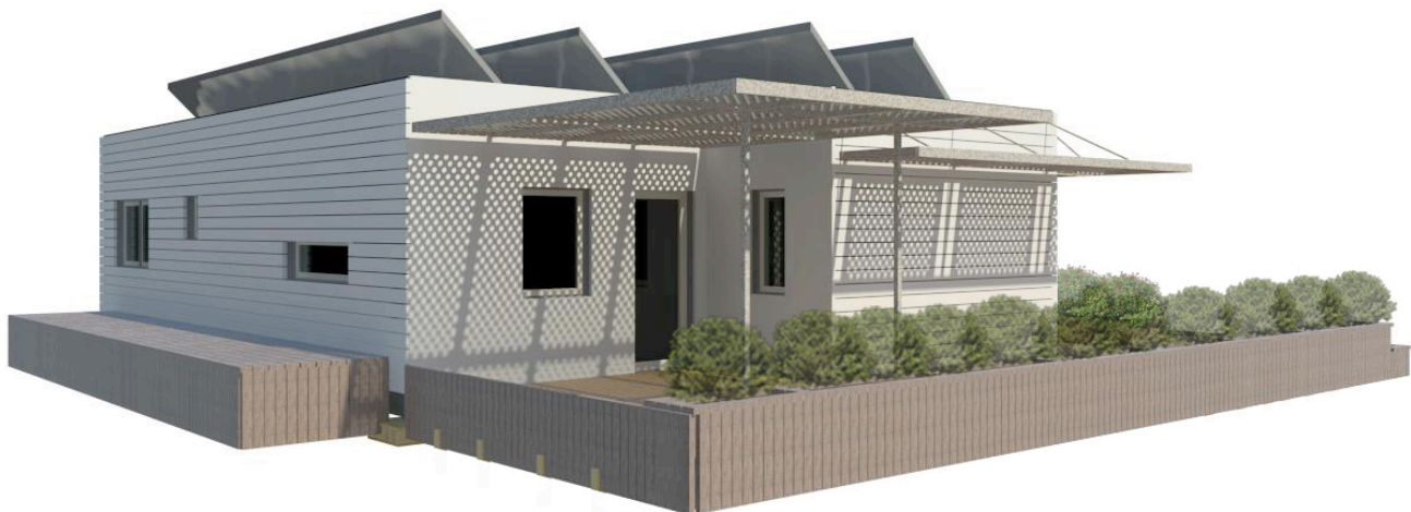
Figure A6: Shading devices along West facade
