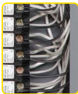
▲ Pigtail Neutral connection
