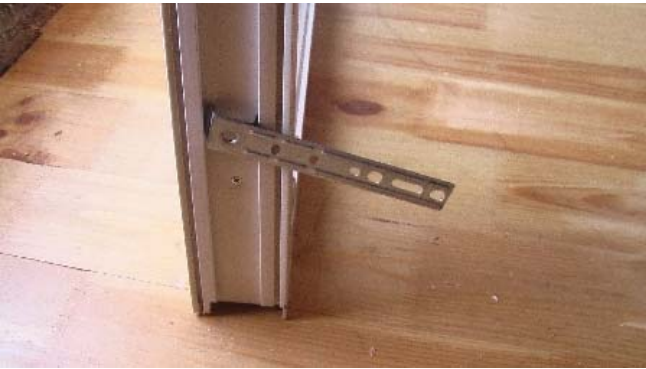
Secure brackets with screws to the frame
