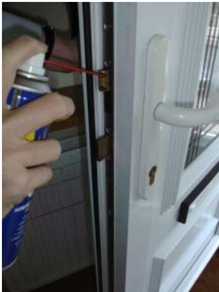
Spraying a door lock
