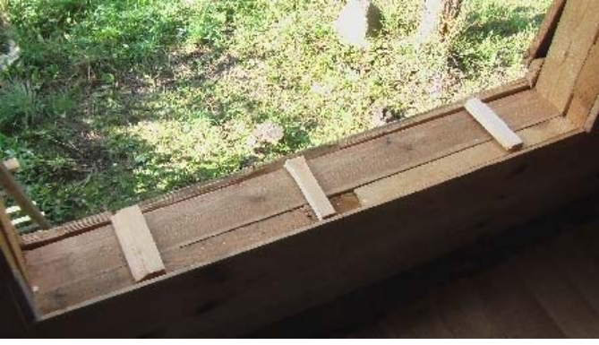
Level the lower part with wood blocks or shims
