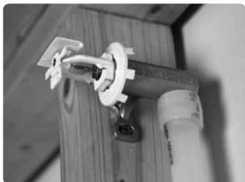
Figure 1-4: ProPEX Elbow with HSW Sprinkler Head
