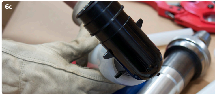
ProPEX Fitting Inserted into 2" Uponor PEX Tubing
