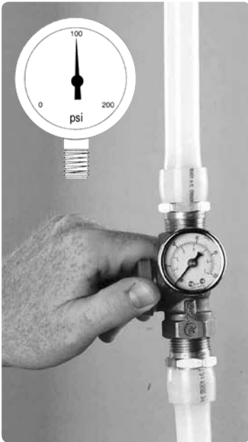
Figure 8-1: Pressure Test at Normal Operating Water Pressure
