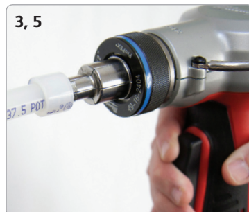
Expansion with Milwaukee M12 ProPEX Expansion Tool
