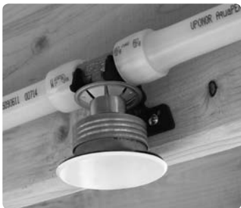
Figure 1-3: ProPEX Tee with RFC Sprinkler Head
