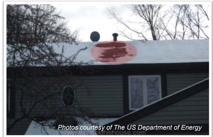
Increases heat loss/gain, and can cause ice dams.
