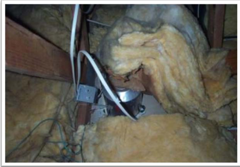
Leaky recessed lighting fixtures...
