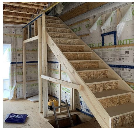
Figure 11: Air barrier lining interior
