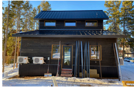
Figure 18: SPARC House after completion of the roof
