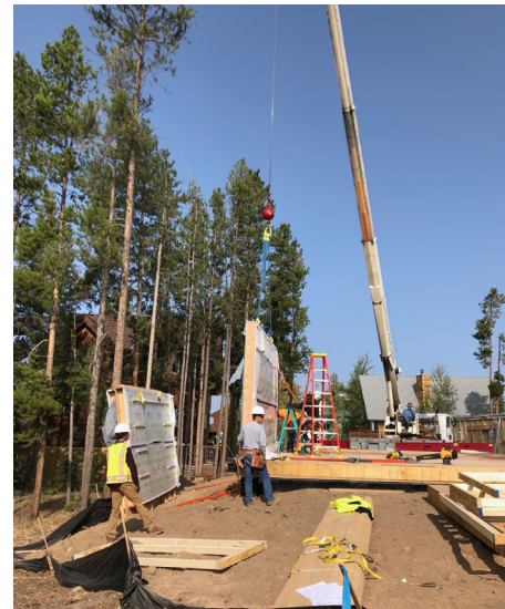
Figure 8: Crane placing panel on floor box
