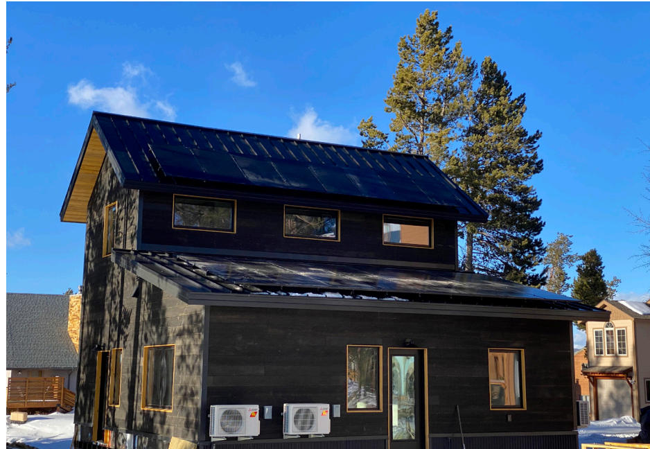
Figure 4: SPARC House showing roofs, PV, and outdoor minisplit units
