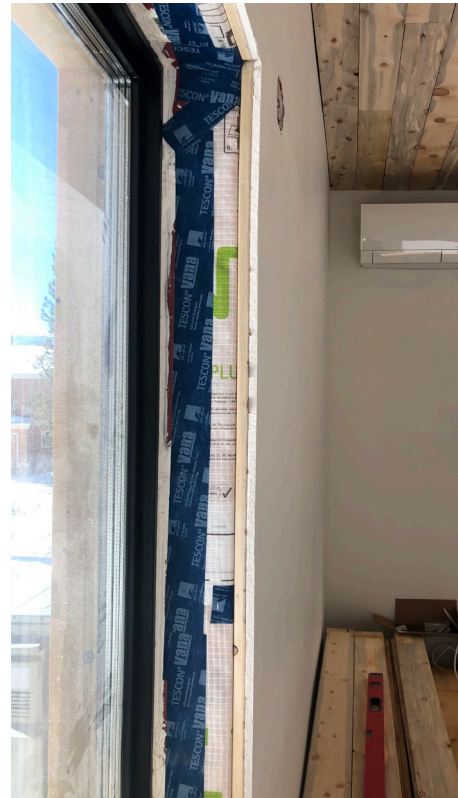
Figure 10: In-set window and wall layers
