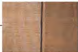
Leading Brand Oil Stain WoodScapes® "after 5 years of exposure"
