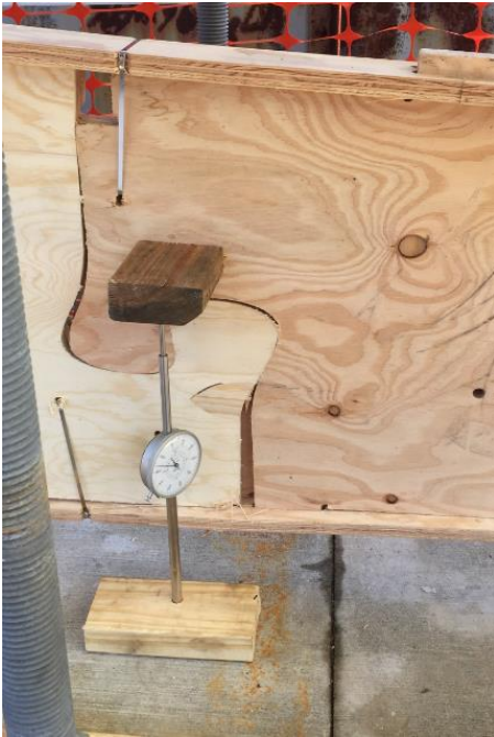
Figure 26: Failure in S-joint
