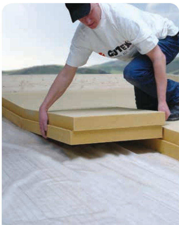
GUTEX Thermoflat® over a concrete substrate
