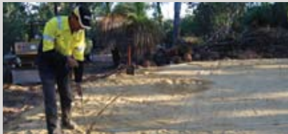
Marking out the tank diameter
