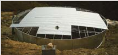
Laying and fitting on the roof sheets across the truss
