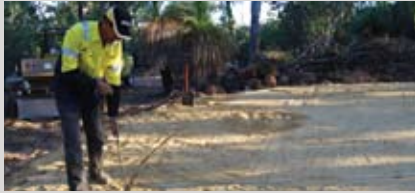
Marking out the tank diameter
