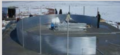
Completion of the first ring
