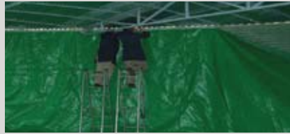
Fitting on and securing the flexible liners
