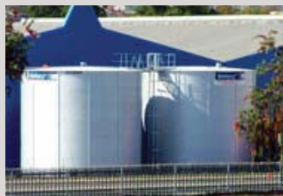
Industrial water supply
