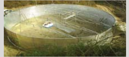
Fitting on the dome truss
