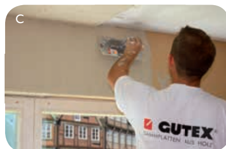
C Apply the plaster over the board
