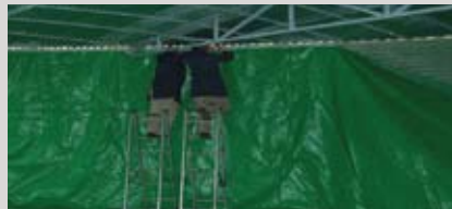
Fitting on and securing the flexible liners
