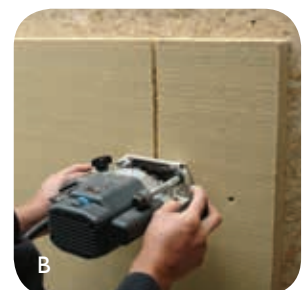
A Fastening GUTEX Thermostat® B Cutting the channels for the service lines C Fastening the gypsum board
