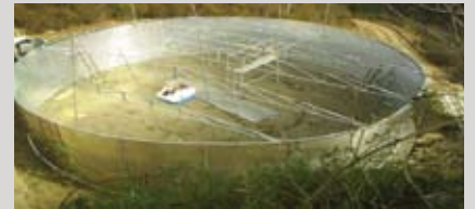
Fitting on the dome truss
