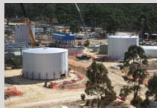
Water supply for mining
