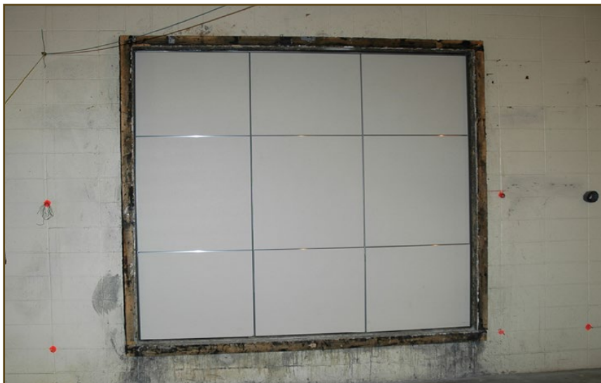
Figure 3. DIRTT walls installed to fill chamber to chamber opening
