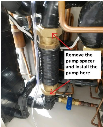
Removing the shipping spacer
