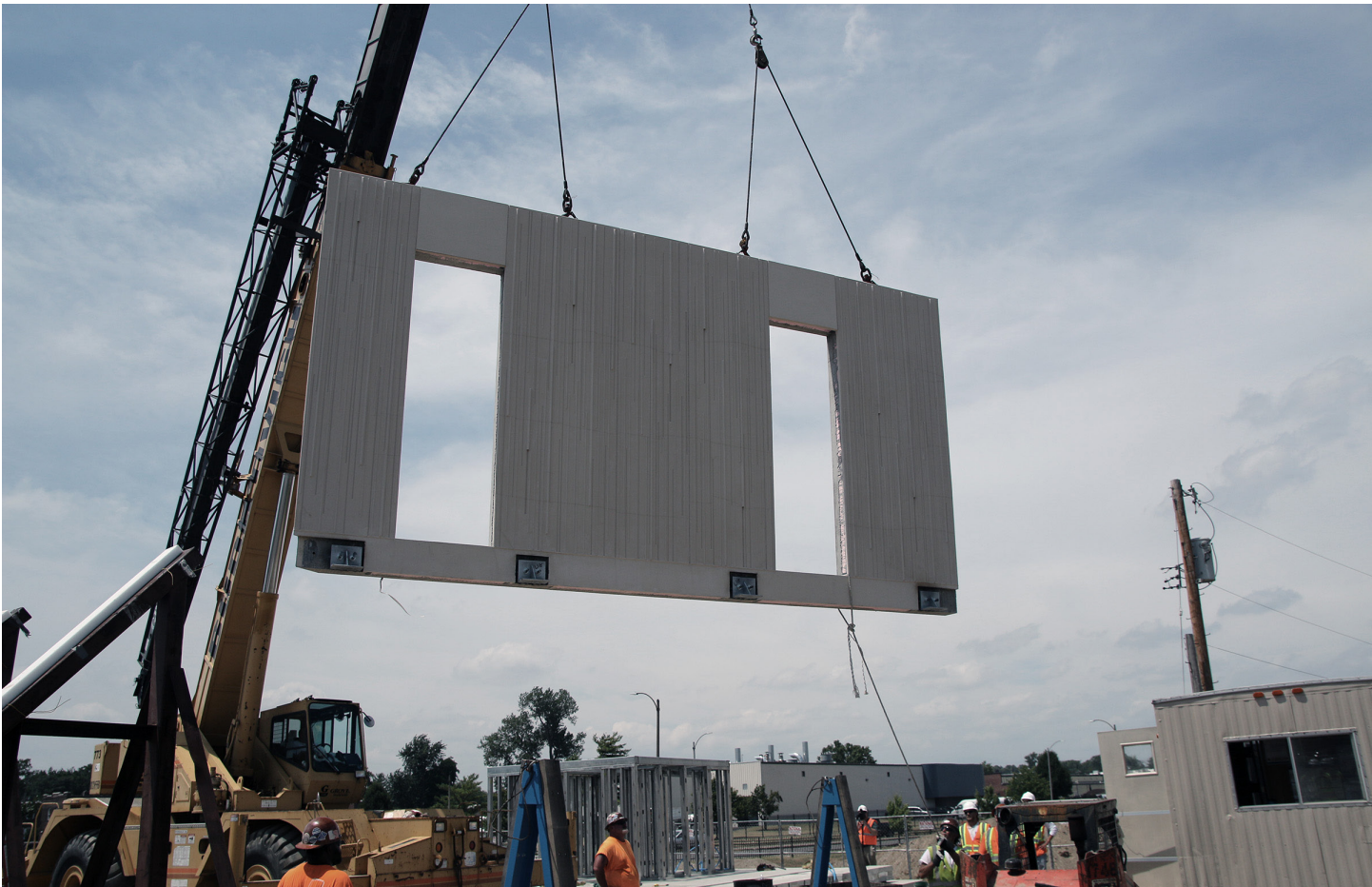
PERECTING PRECAST WALL PANEL
