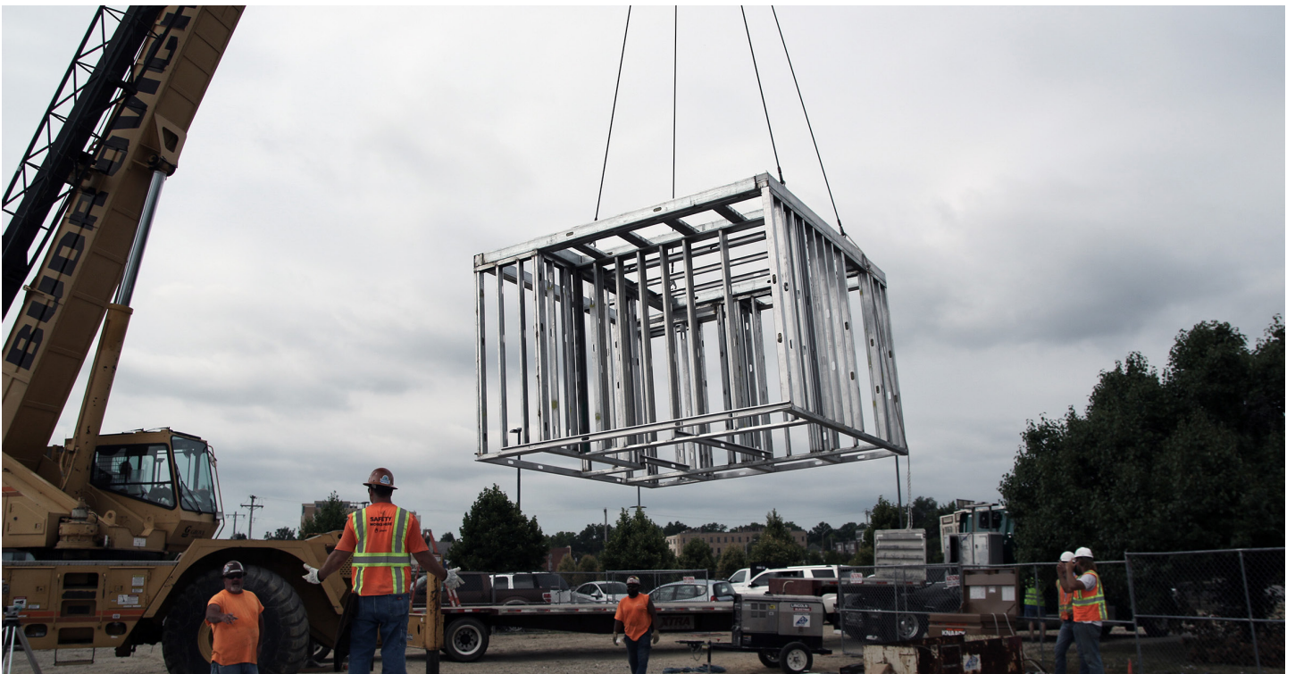
PLACING LIGHT GAUGE STEEL CORE
