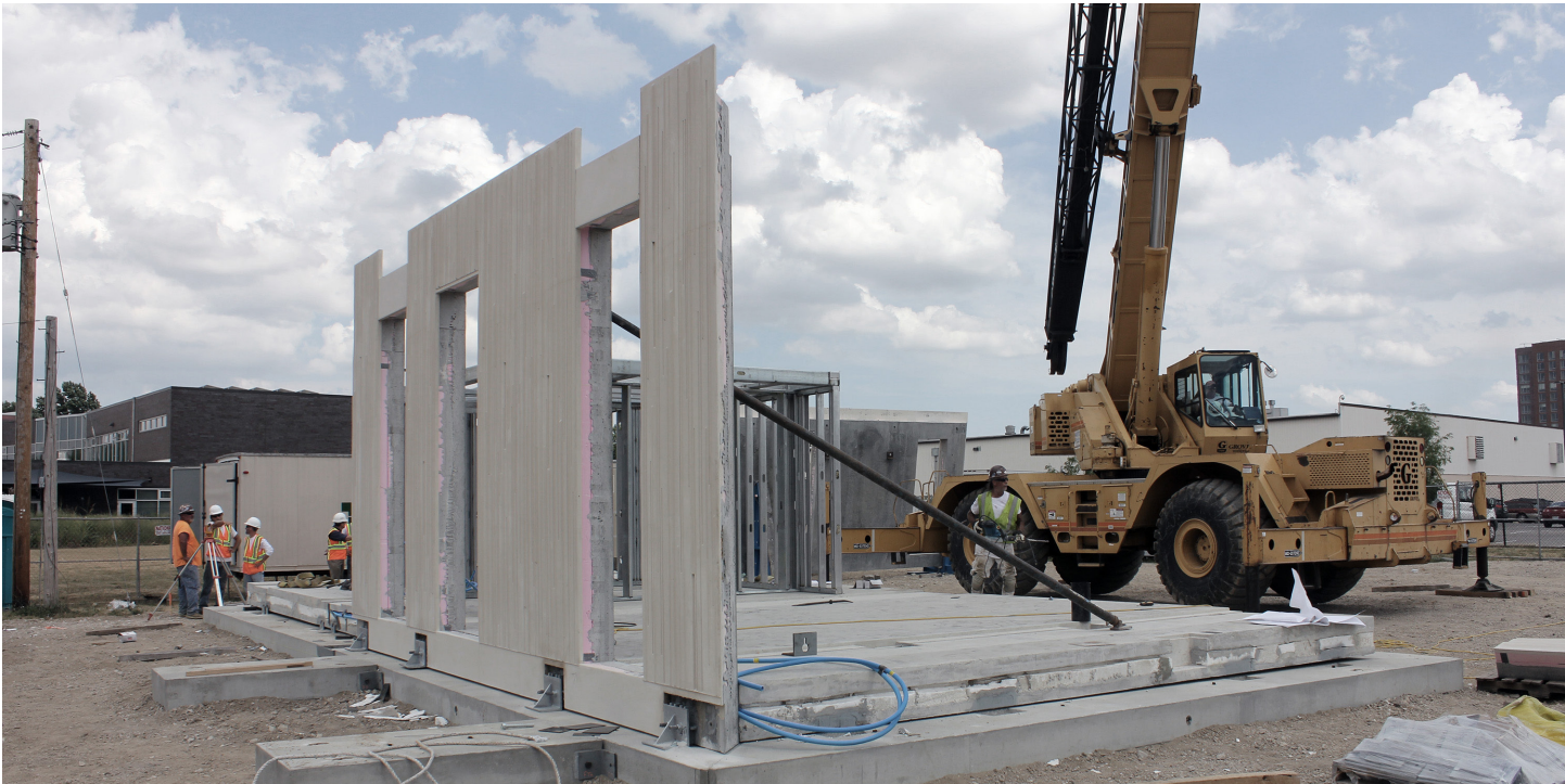
BRACING FIRST PRECAST WALL PANEL
