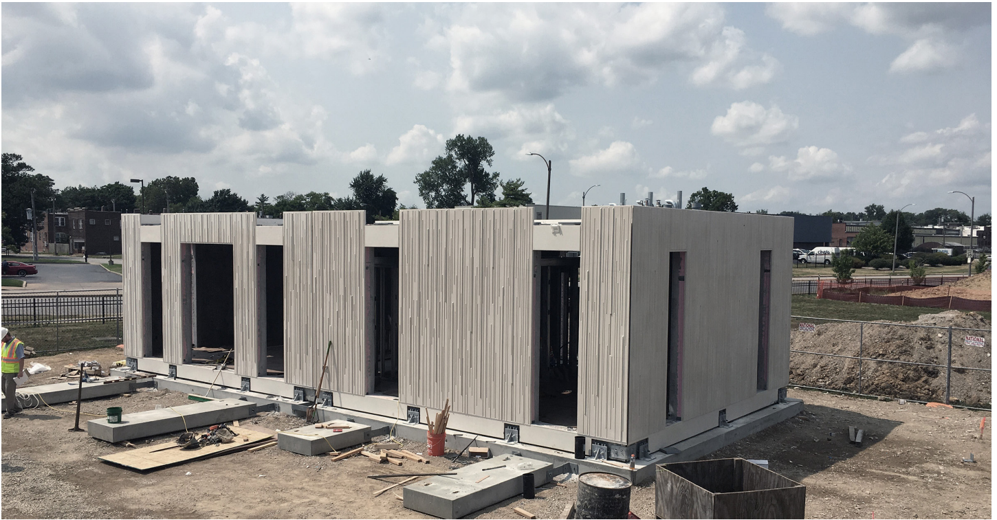
PRECAST ENVELOPE ERECTED
