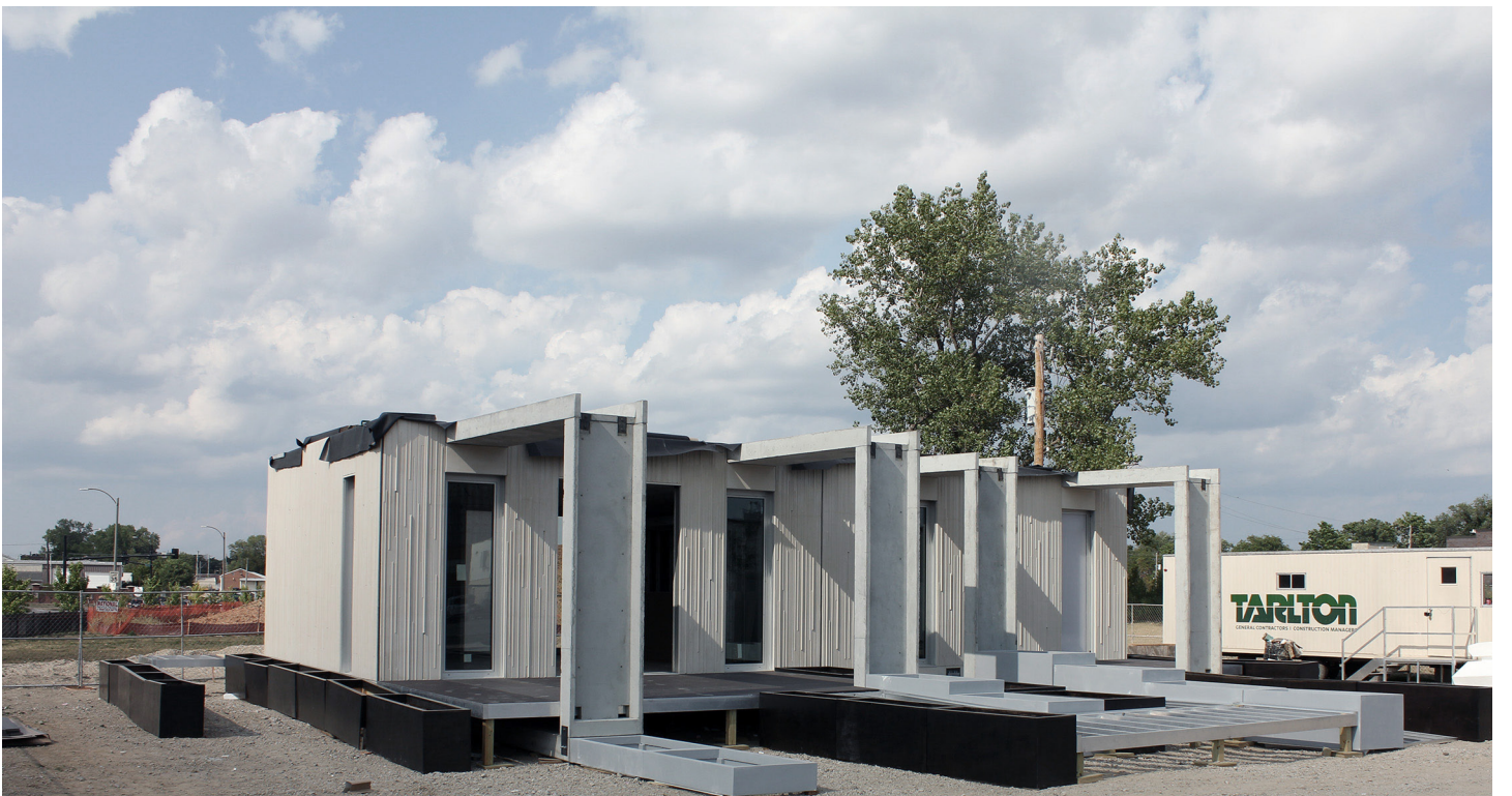
CRETE house IN PROGRESS
