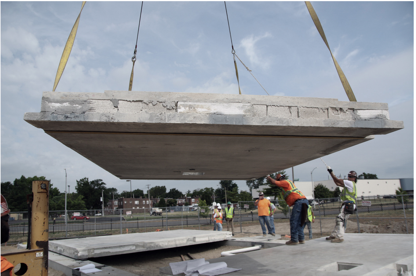
PLACING PRECAST FLOOR SLABS ON SITE
