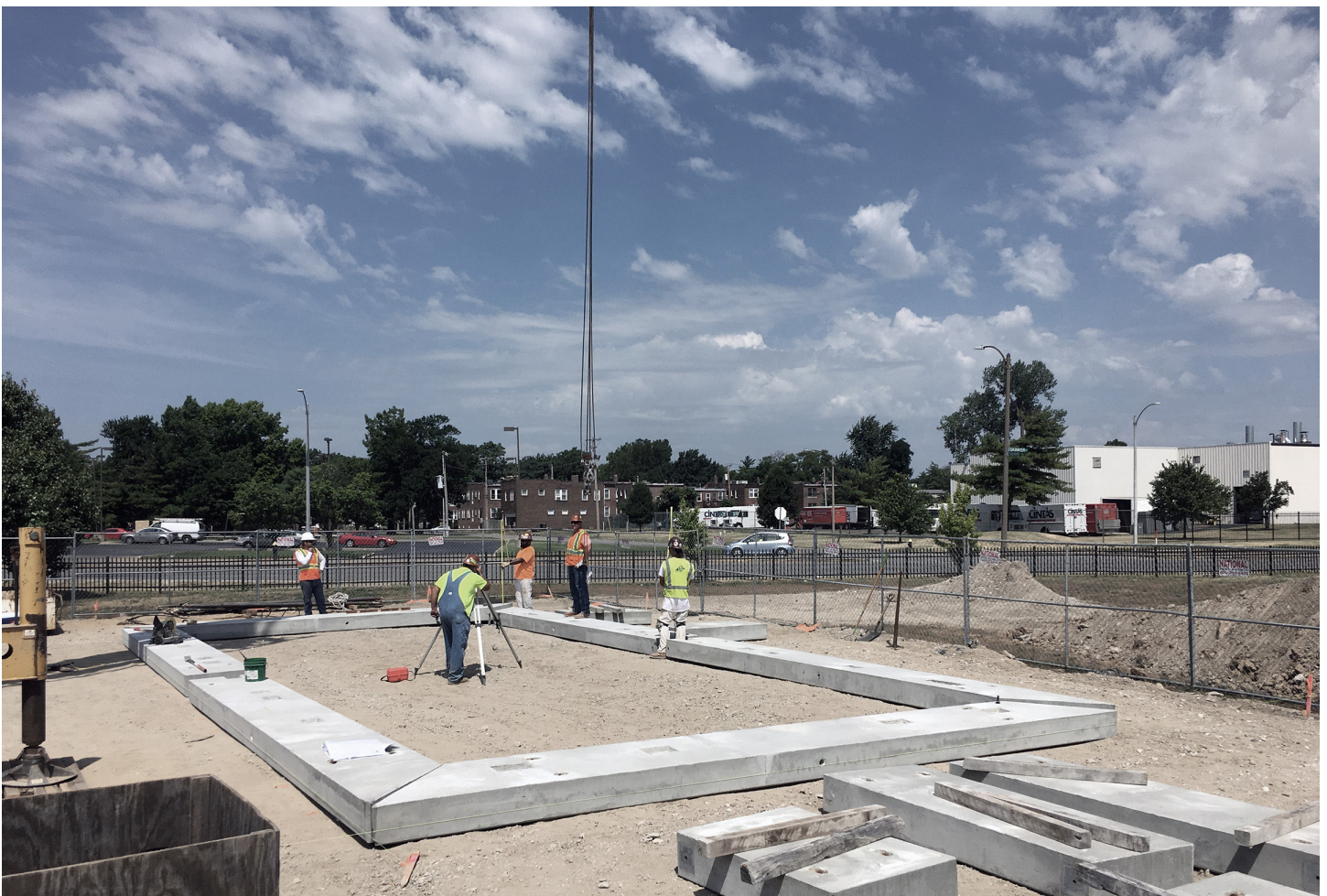
PLACING FOOTINGS ON SITE
