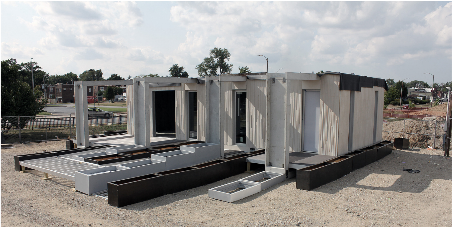
CRETE house IN PROGRESS
