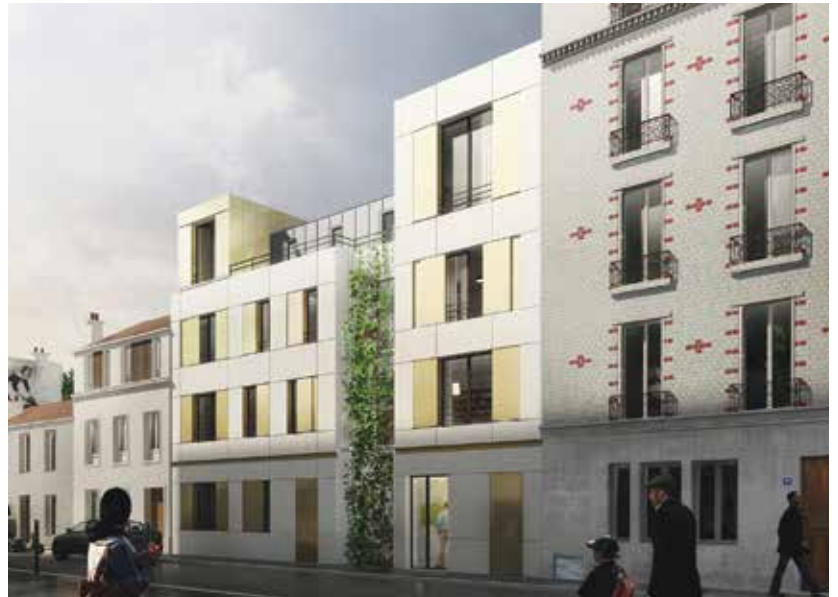
Stone-like cladding that fits seamlessly into the street facade, Paris, France.
