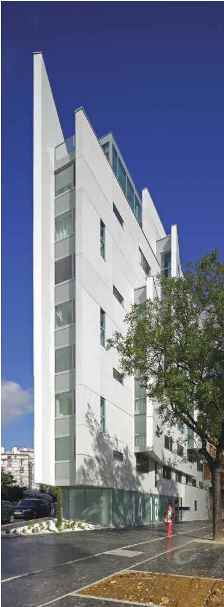
Ductal® facade panels for a narrow, ten-story student residence building on a triangular site - Paris, France.
