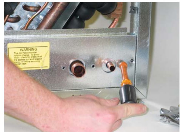
Remove side panels as shown.
