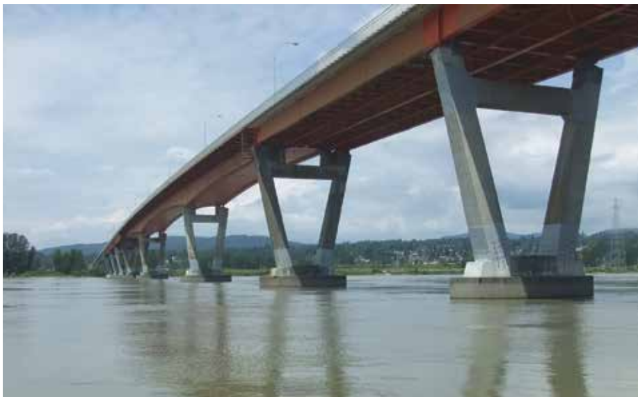
Mission Bridge - Before: two columns to be retrofitted. Ductal® was delivered onsite in ready-mix trucks. After: completed columns with Ductal® jacket - British Columbia, Canada.
