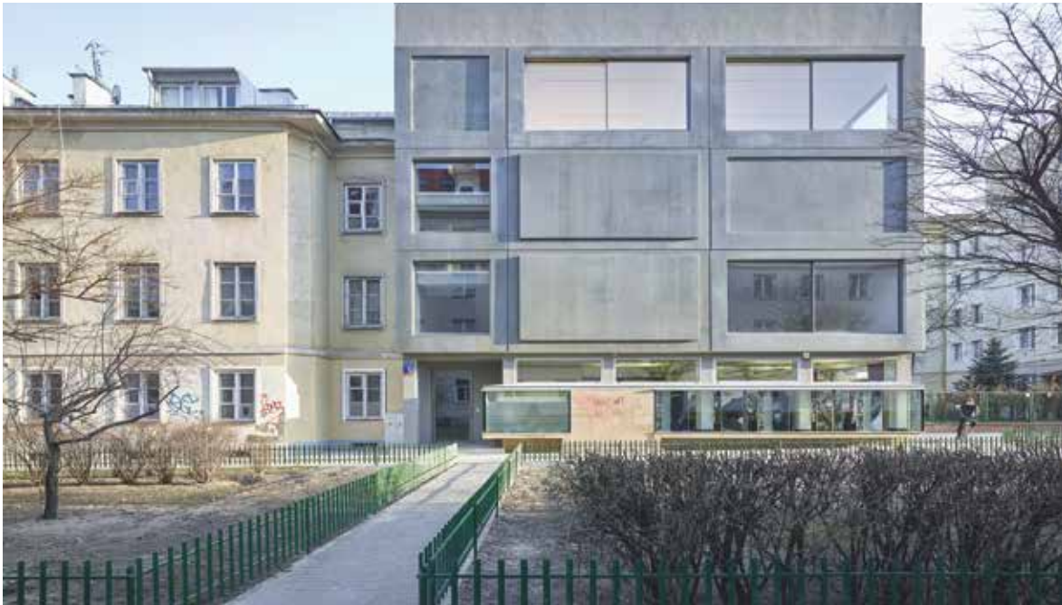
Foksal Gallery Foundation: a return to the mineral appearance of exposed concrete – Warsaw, Poland.
