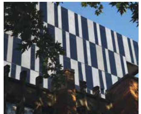
Ductal® panels contrast with glazing at the Rotman School of Management - University of Toronto, Canada.
