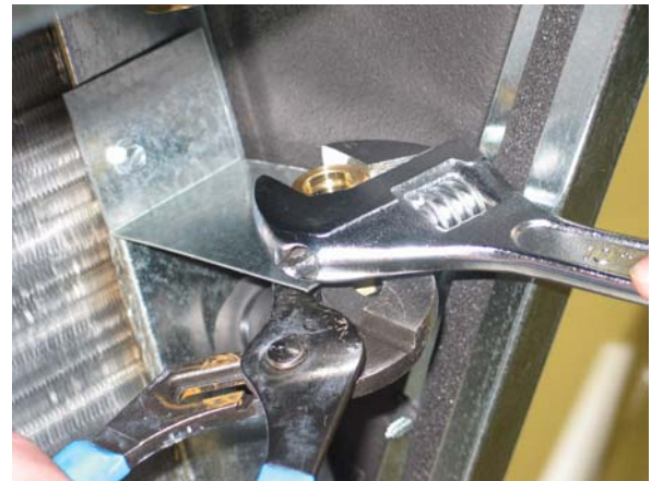
Remove nut as shown.
