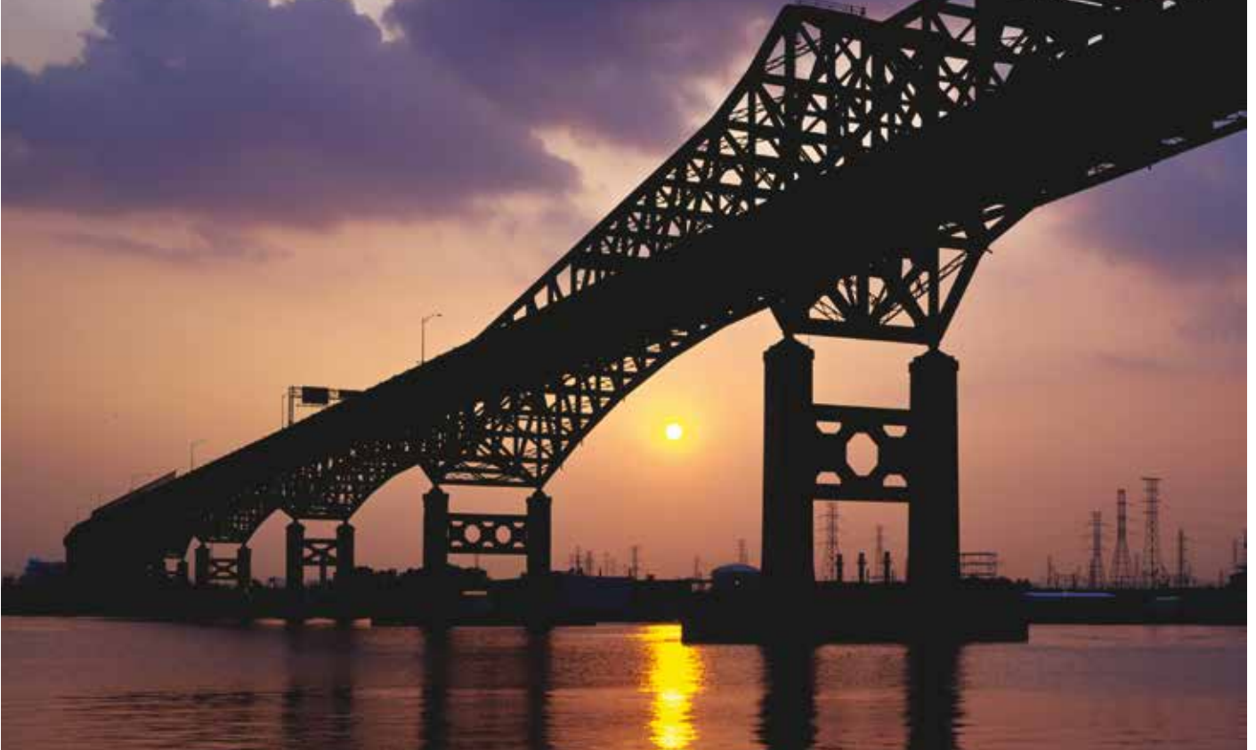
The Pulaski Skyway Rehabilitation project in the United States was the first in North America to place Ductal® joint fill by concrete pump. The material flowed continuously along a pipe 170 m long and 7.5 cm in diameter.
