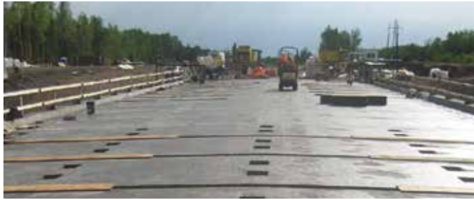
A precast bridge deck ready for joint fill.
