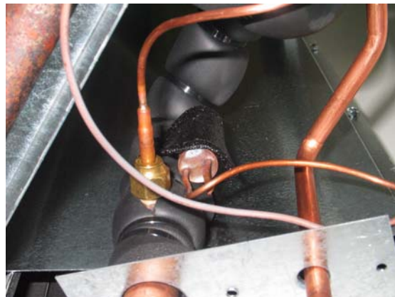
Secure bulb with cork tape as shown.
