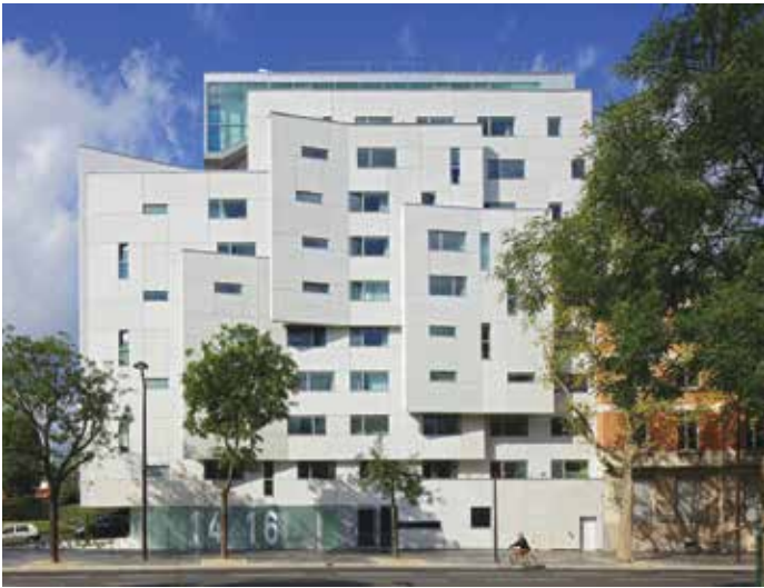
A 65-room student residence designed by Jacques Ripault Architecture.
