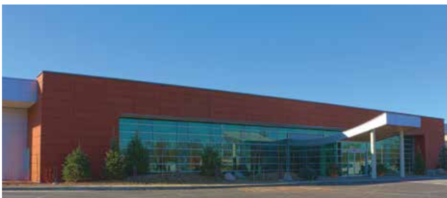
Thin Ductal® panels create an attractive cladding solution for the new Rosecrance Ware Center - Rockford, Illinois, United States.
