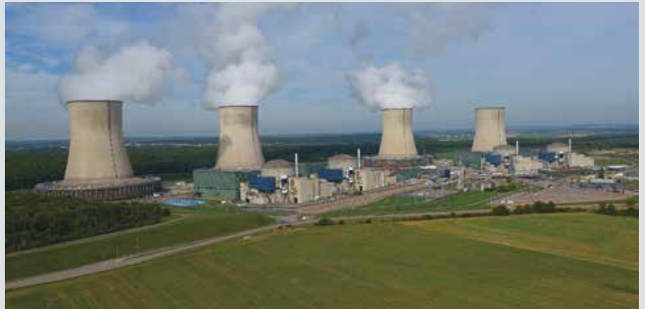
The Cattenom Nuclear Power Station - Moselle, France.
