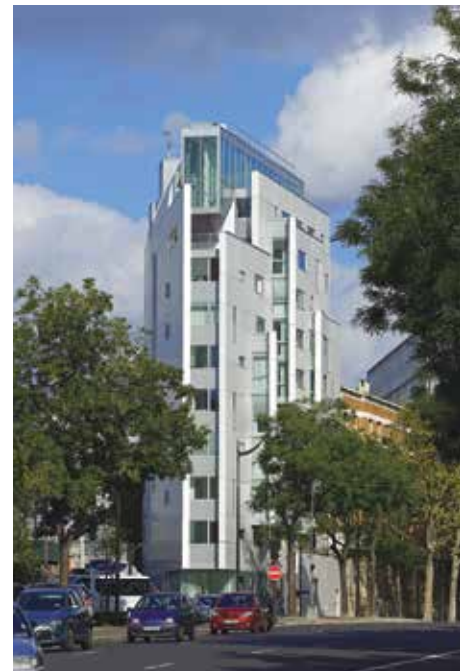
Facade panels provide external thermal insulation - student residence, Paris, France.
