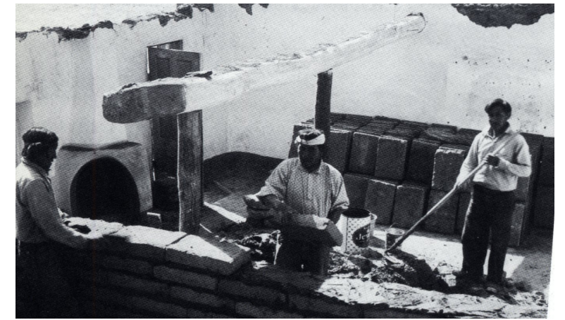
Hopi men assembling a sandstone wall.
