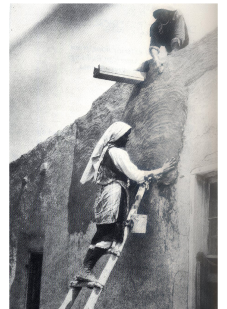
Hopi woman applying plaster to sandstone wall.
