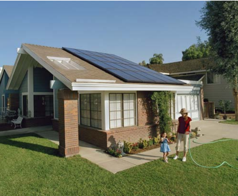
A BP Solar energy system of about 3.5 kW helps power this home in California.
