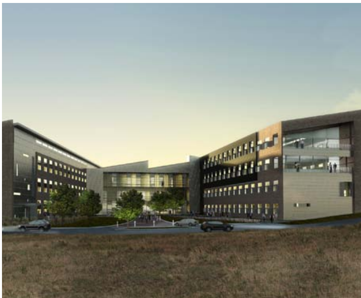
NREL's Research Support Facilities, scheduled for completion in the summer of 2010, will house 740 NREL and U.S. Department of Energy staff members. (NREL PIX 16250, RNL Design)
