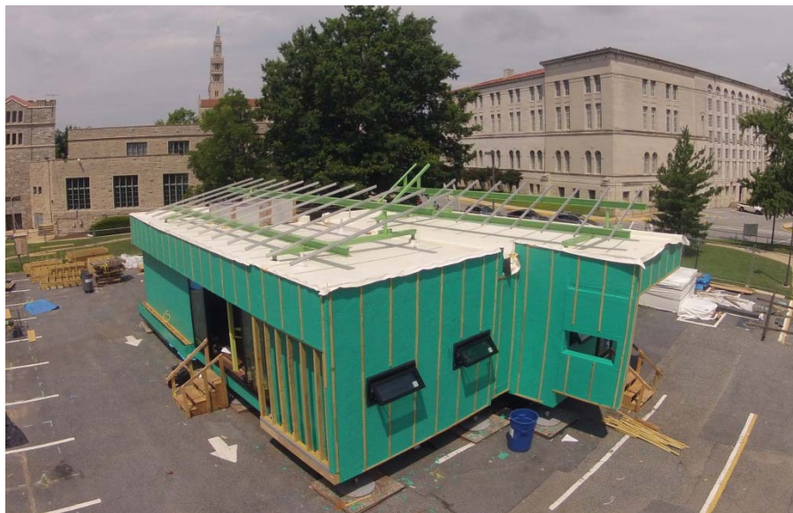
Construction Photo Showing White EPDM Roof Membrane
