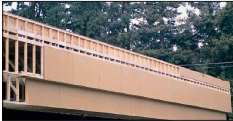
MDO panels create a smooth, easy-to-finish surface in fascias.
