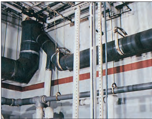
Harvel CPVC piping can be integrated into hot corrosive drainage systems.
