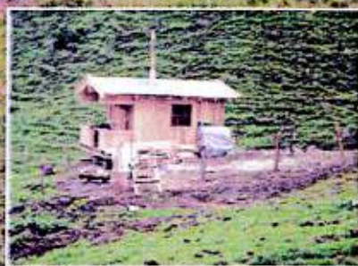
The finished structure.
