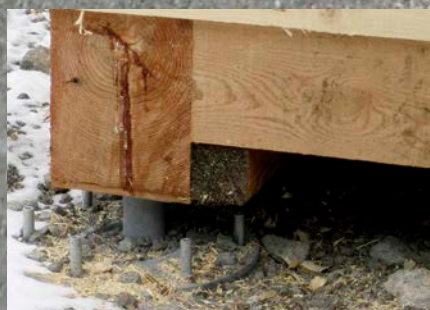
Spider anchor XII as foundation for a year-round occupied single-family house, Salzburg (A)
