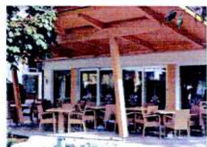
The finished construction. Terrace roofing, Maishofen (A)
