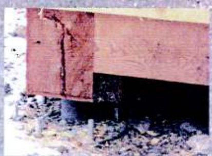
Spider anchor X1 as foundation for a round occupied single-family house, Salzburg (A)
