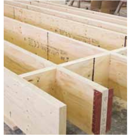
Pre-assembled box girders for roof construction.
