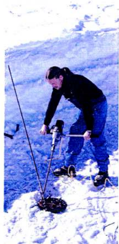
The spider anchor (System version 1.1; 2007 – 2011) achieves a high level of load-bearing capacity not only in cohesive and non-cohesive ground but it is also highly suitable for safe and secure anchoring of heavy loads in ice and snow.
