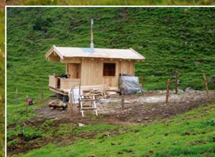
The finished structure
