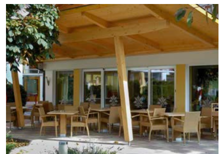
The finished construction. Terrace roofing, Maishofen (A)
