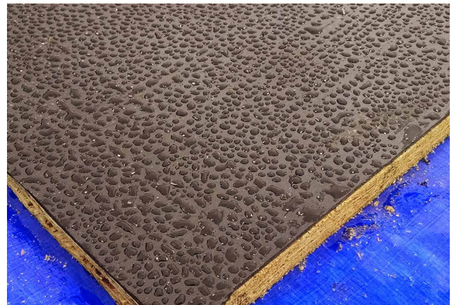
A high strength ABS layer is laminated to typical OSB floor sheathing. Once the seams are bonded, this creates a strong, waterproof shell underneath the home.
