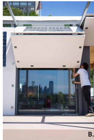
East, west and north-facing facades of the SURE HOUSE are covered with traditionally-inspired cedar shakes (A) while the south side of the home is comprised of extra large high-performance windows secured with a state-of-the-art innovative fiber composite storm shutter system (B) .
