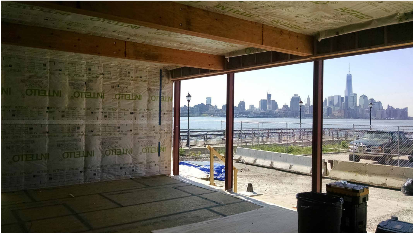
FIGURE 3D-4: LIVINGROOM AIR SEALING
