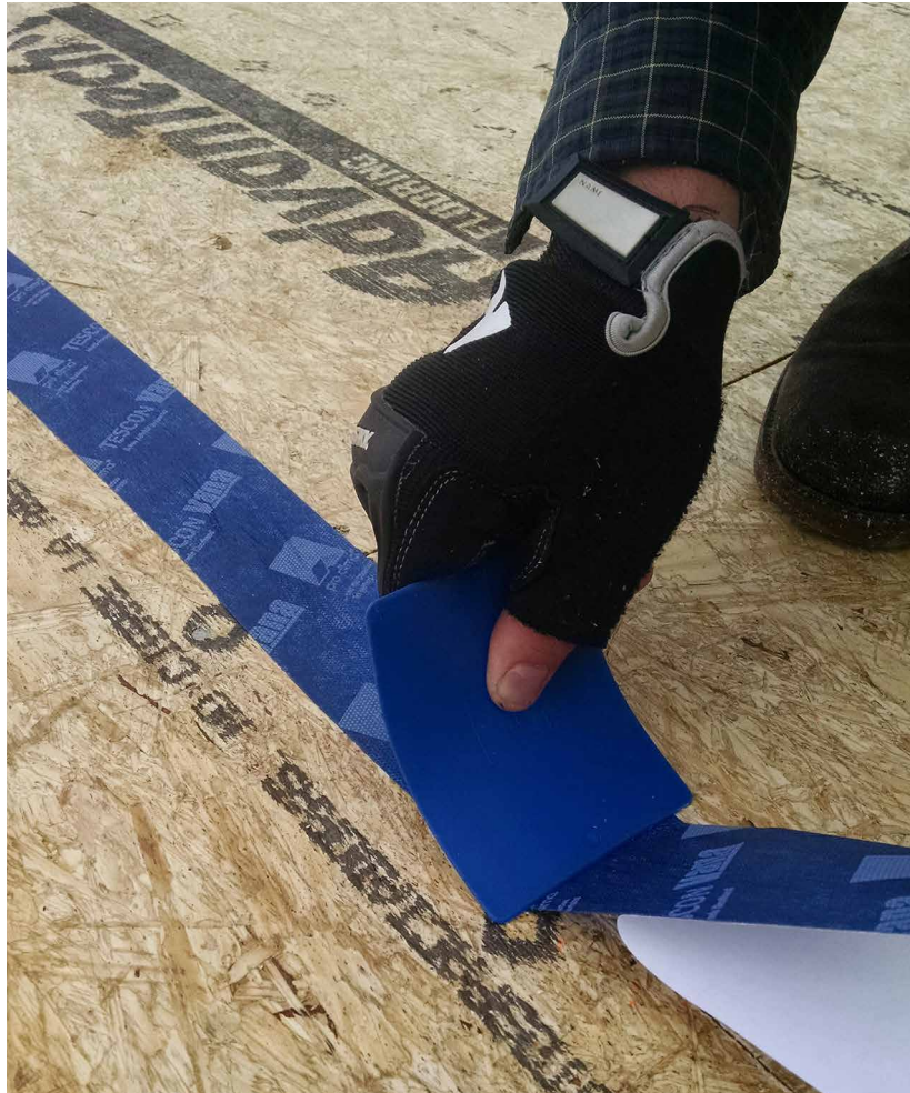
FIGURE 3D-1: SUBFLOOR AIR BARRIER TAPING DETAIL
