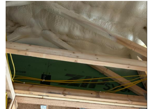
Figure 1: Spray foam insulation and Zip sheathing
