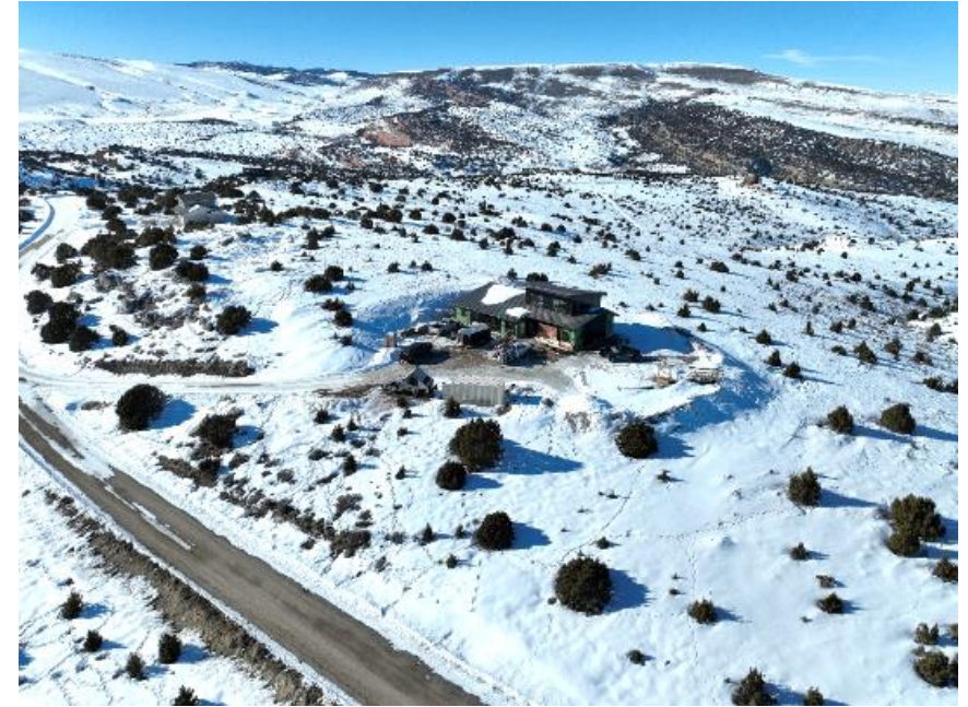
Figure 8: The Wind River home demonstrates the potential for net-zero spec home construction
