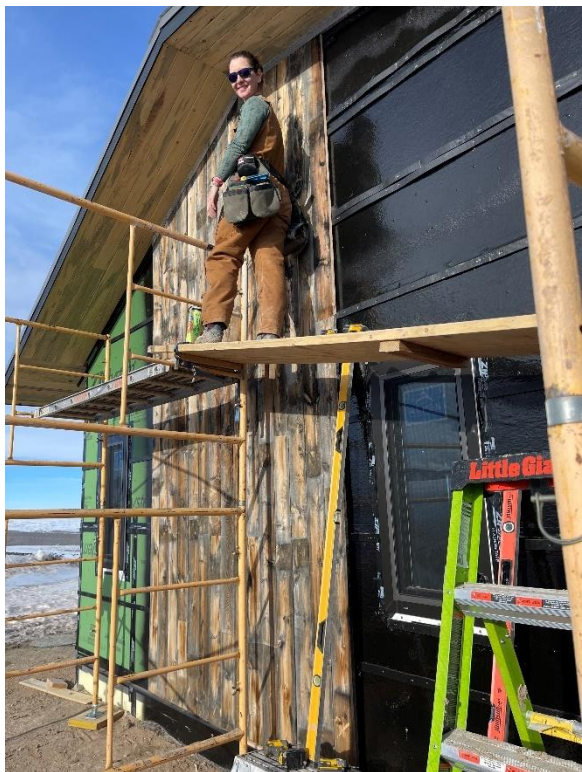
Figure 4: Reclaimed snow fence siding being installed at Wind River home.
