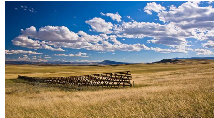
Figure 1: Wyoming snow fence, used to create drifts next to roadways.
