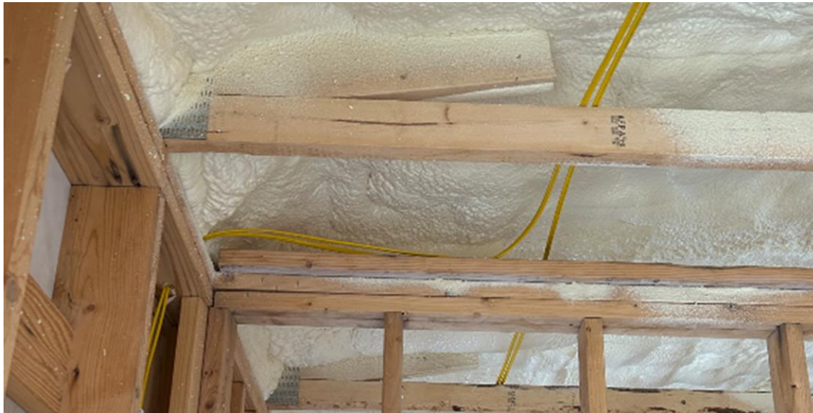
Figure 2. Insulated attic space
