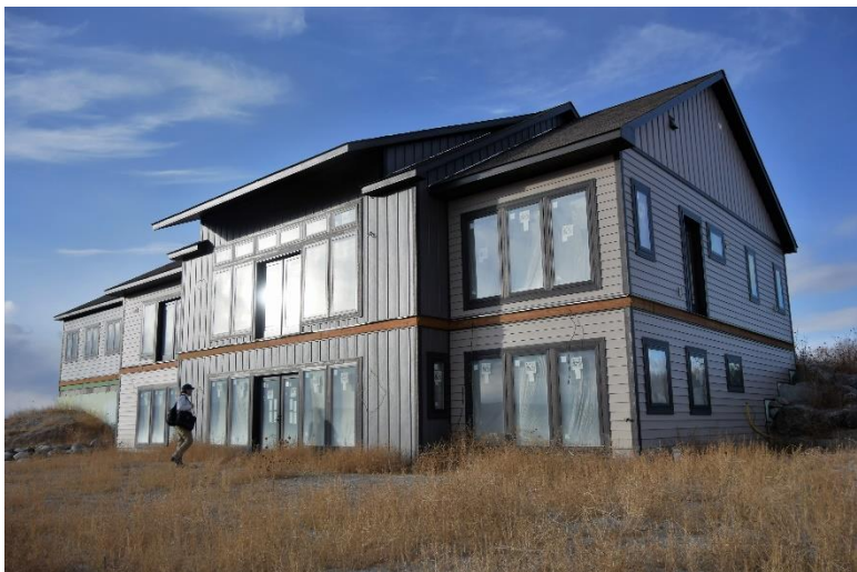
Figure 5. Zero-energy house near Shoshoni, Wyoming, designed by UW faculty lead Jon Gardzelewski, AIA, and built by Timshel Construction.
