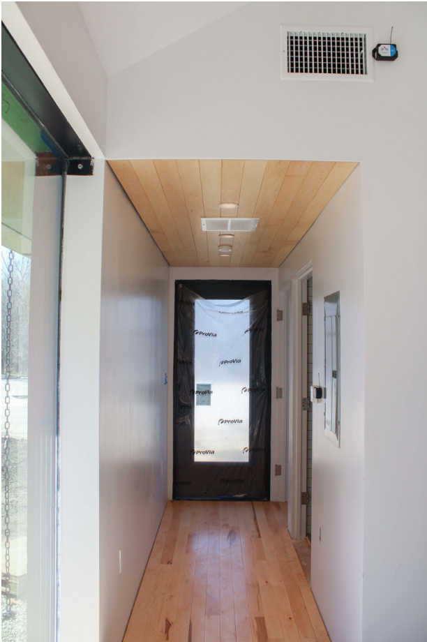
Haven Studio, photo of interior showing the hallway
