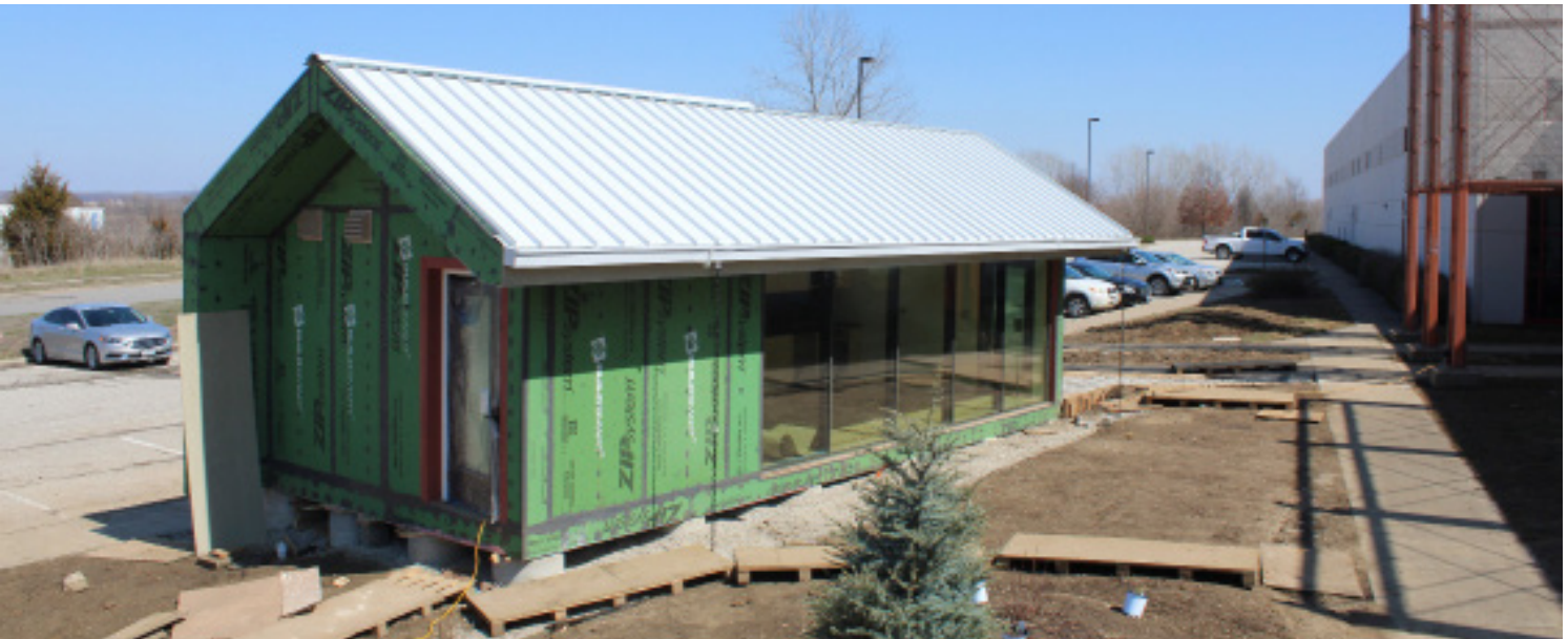
Haven Studio, photo of the south and east facades.
