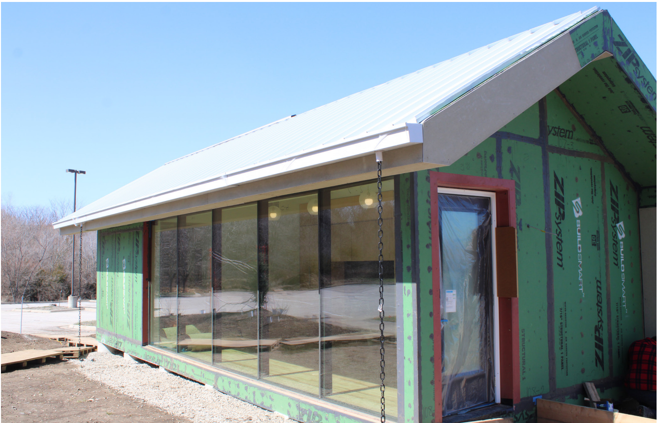
Haven Studio, photo of exterior showing the south and west facades.
