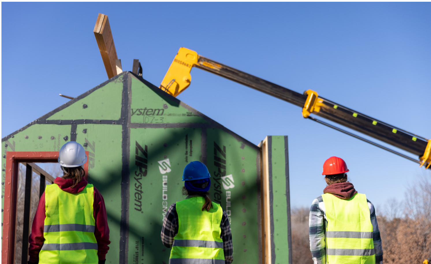
Haven Studio, photo of installing the ridge beam onto the Build SMART prefabricated wall panels.
