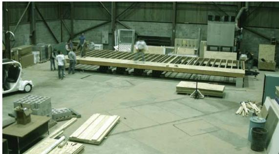
By building the house indoors, we were able to minimize exposure to radon sources in the ground. In addition, a layer of Tyvek, plywood and latex paint was placed below the floor slab in order to eliminate moisture radon penetration during the shipping of the house to and from Washington, D.C., and to prevent radon gas from being absorbed into the house after the competition.
